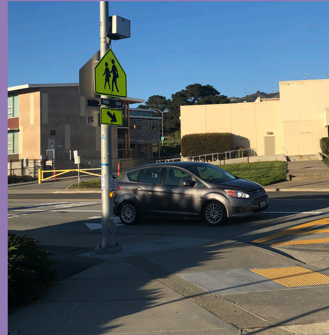
RECTANGULAR RAPID FLASHING BEACON
