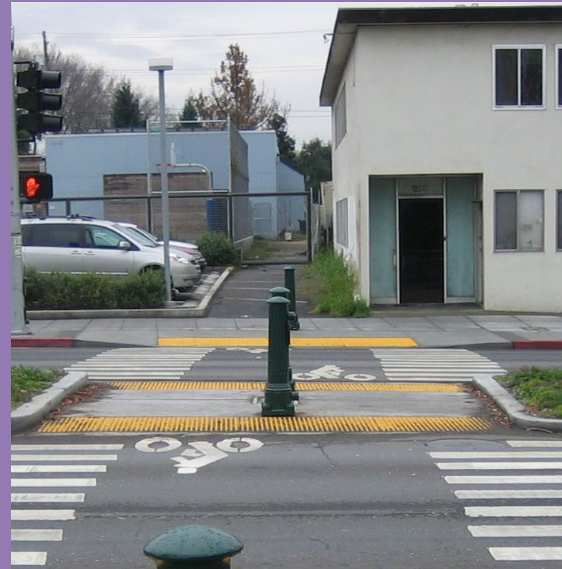
MEDIAN ISLAND REFUGE
